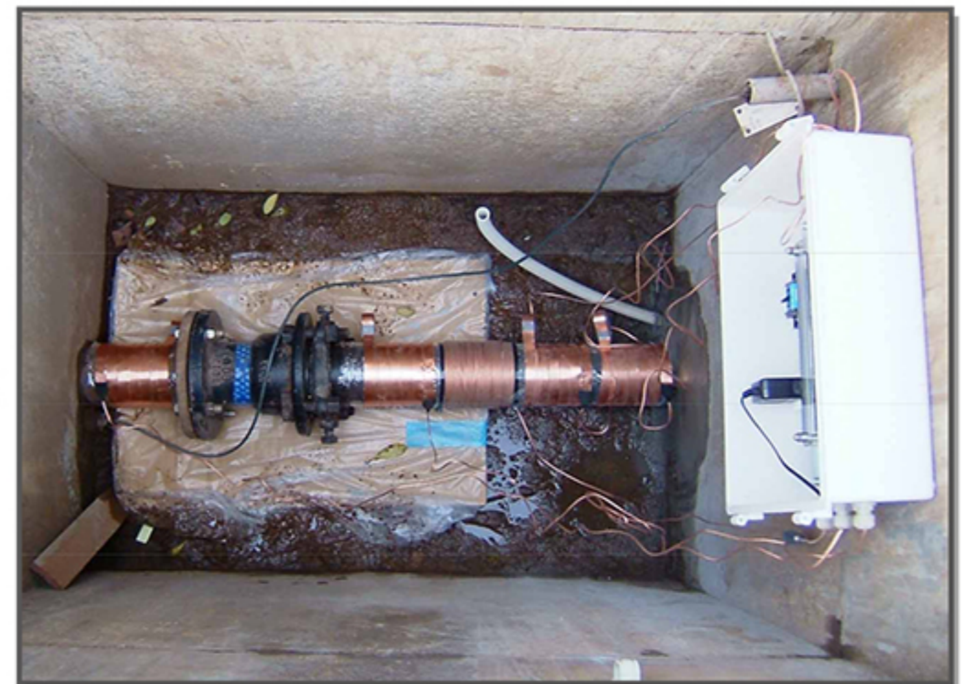
[Cable winding completed]
