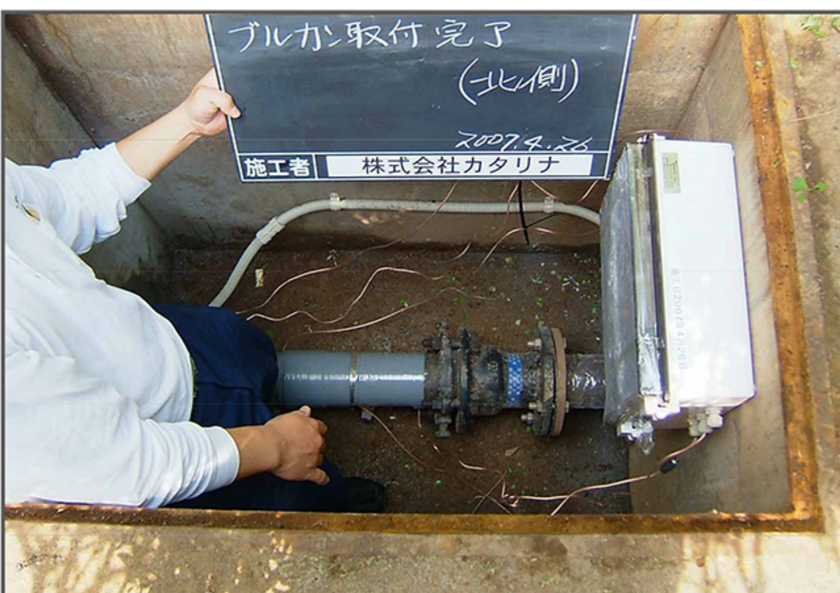
[Installation of the Vulcan completed]
