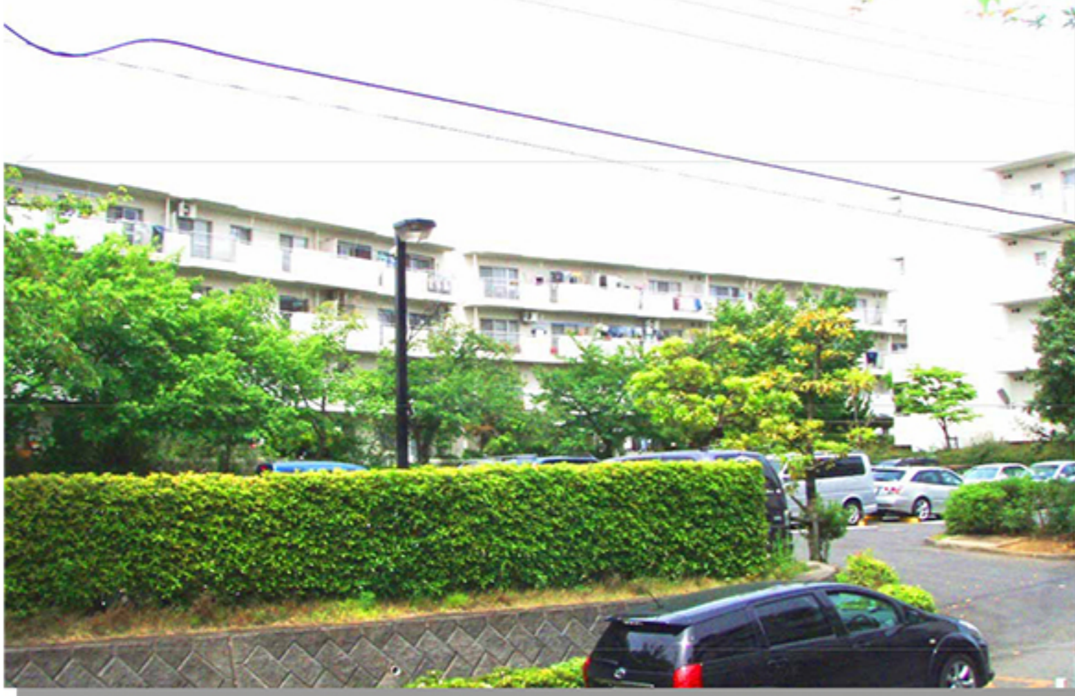
[Overall view of the apartment building]
