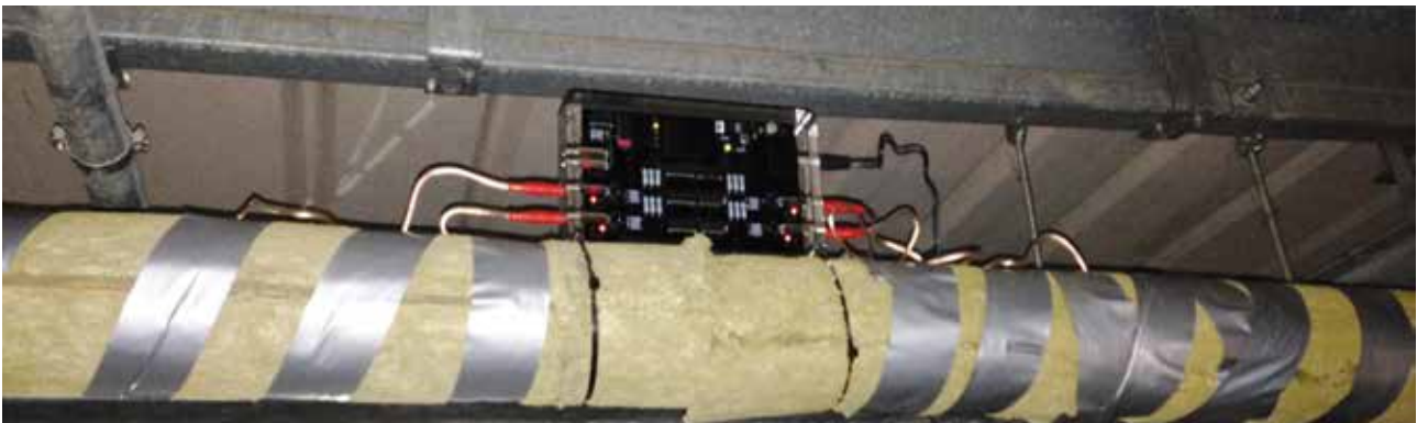
Vulcan S25 unit installed with insulation re-wrapped over the pipes and impulse cables
