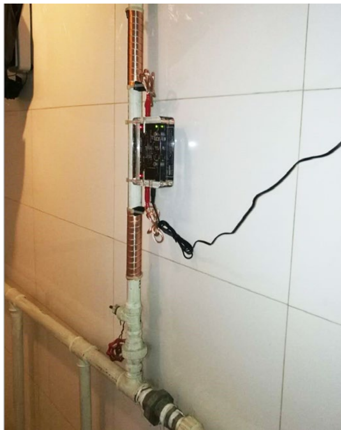
Vulcan 3000 was installed on a solar water pipe to solve the scaling problem of the solar vacuum tubes.
