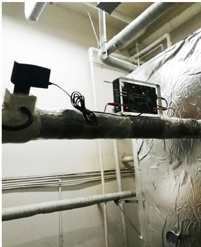
Vulcan S10 was installed in front of the heat exchanger to solve the scaling problems of heat exchangers, pumps, water tank, shower heads and the whole piping system.
