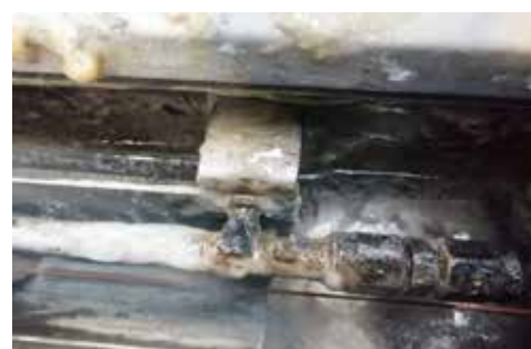
June 13 : Vulcan had been removed for 1 month. The Machine 1 has returned to its initial state, floating with biofilm.
