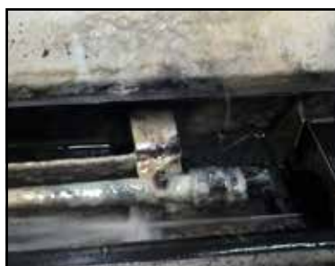
February 07 : Visual observation of the Machine 1 before Vulcan was installed. The wall and the nozzles have scale and bacteria.
