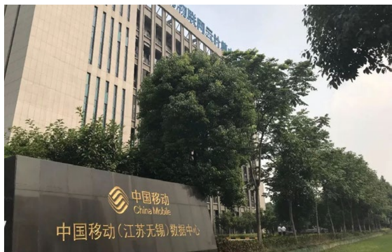
China Mobile data center (Jiangsu Wuxi)
