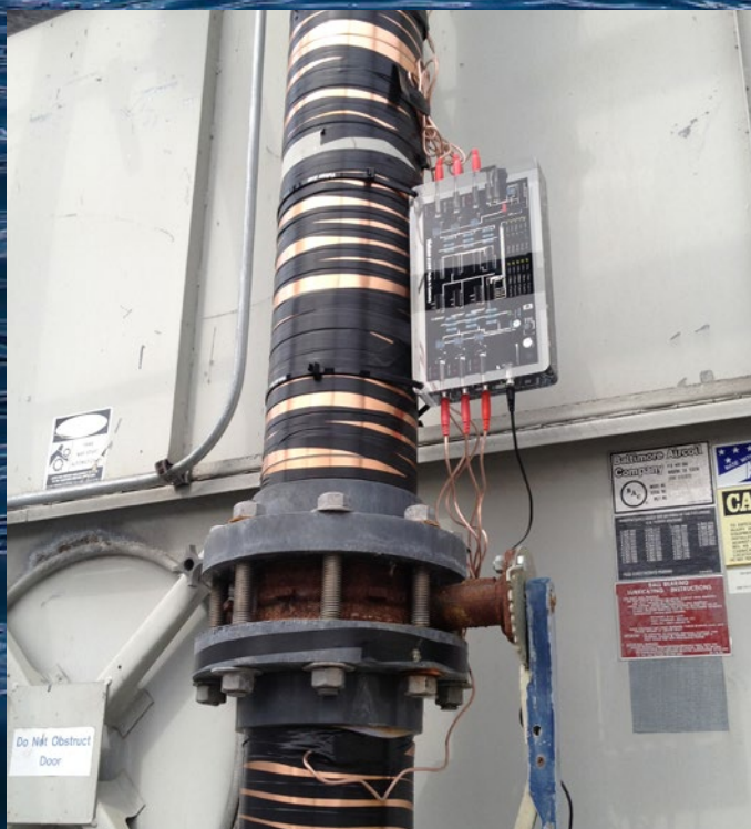
Vulcan S100 installed on cooling towers
