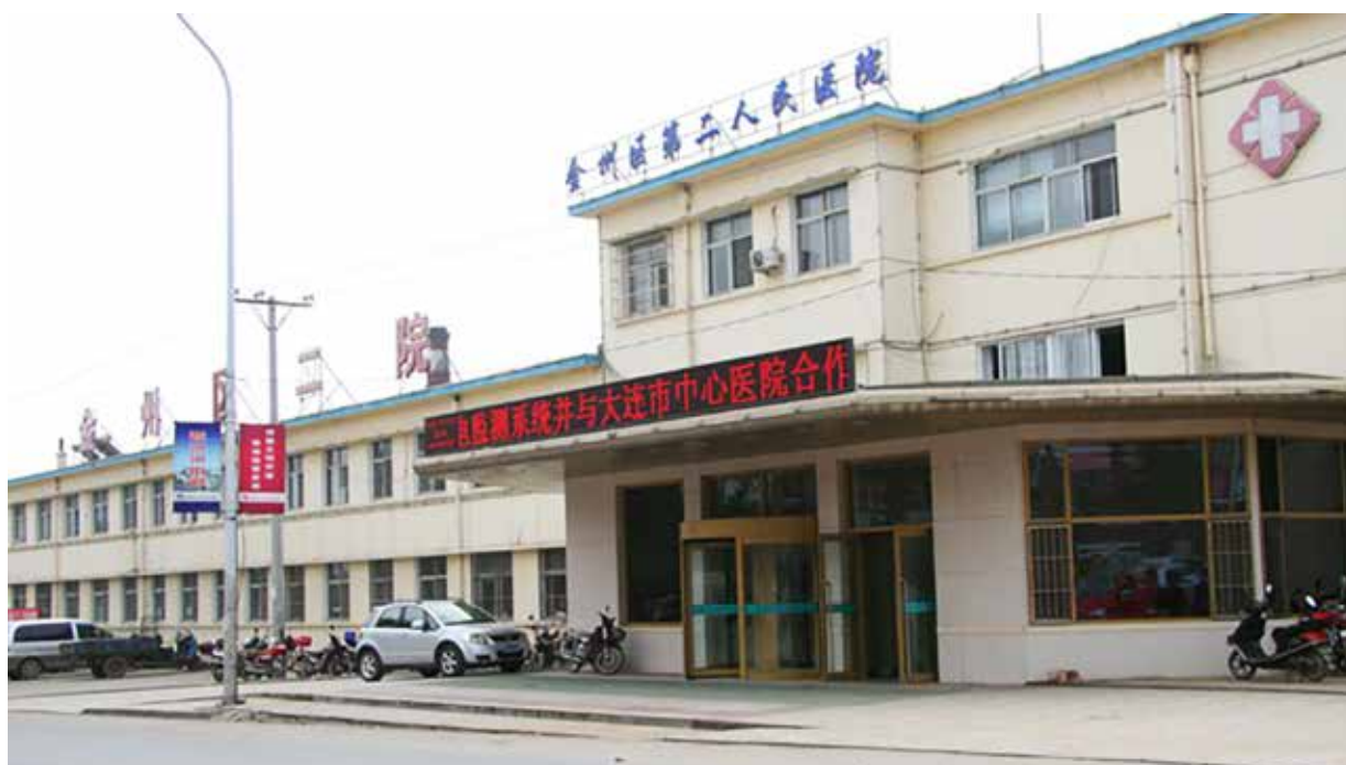
The front door of Jinzhou No.2 People's Hospital in Dalian city.
