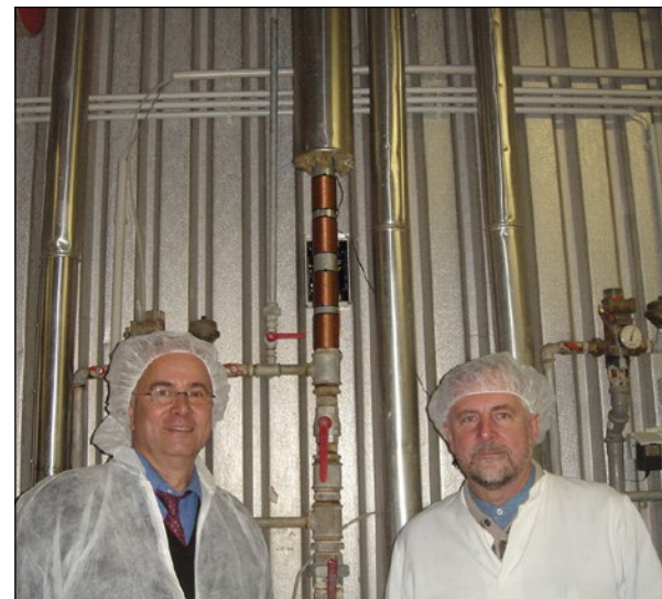
Mr. Christiani at installation of Vulcan
