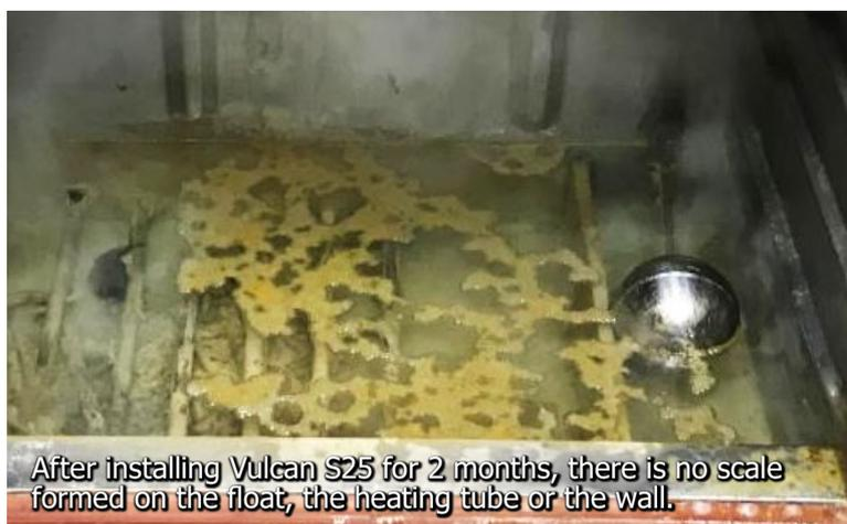
After installing Vulcan S25 for 2 months, there is no scale formed on the float, the heating tube or the wall.
