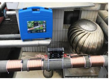
Vulcan S25 was installed on the main water pipe of the guest room Builing B.
