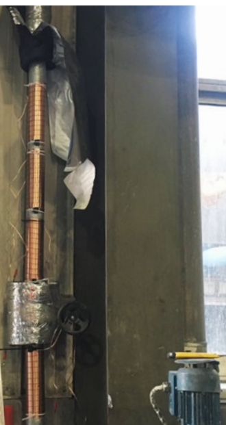
Vulcan S25 was installed on the main inlet of the cooling towers for the molding factory.
