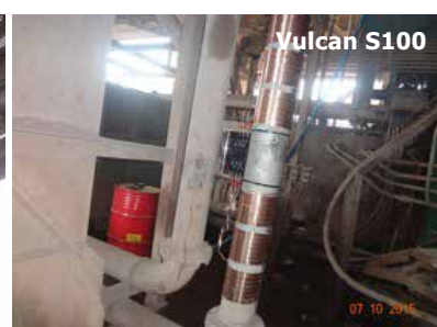
Heat exchanger after 2 months Vulcan installation
