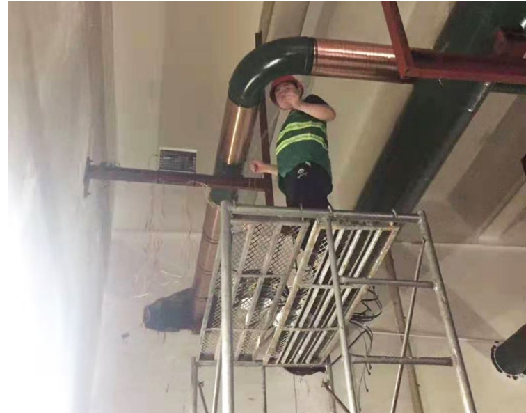
Vulcan S350 was installed on the circulating cooling water pipe for the textile equipment.
