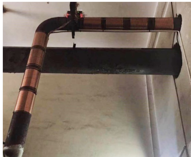
Vulcan S250 was installed on the circulating cooling water pipe for the textile equipment.
