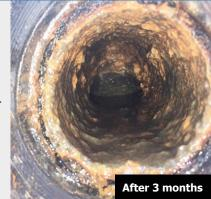
After 3 months the rust in the pipe has lightened and the amount of scale is gradually reducing.
