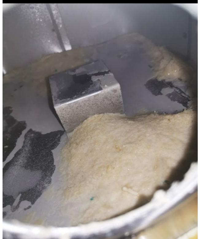
The scale has been completely turned into powder, so there is no need to open it for cleaning, just by operating the regular drainage function, it can keep the hot water tank clean and free of scale. Due to the good results, the cooperation will also be carried out in the hotel's hot water supply system and central air conditioning system.
