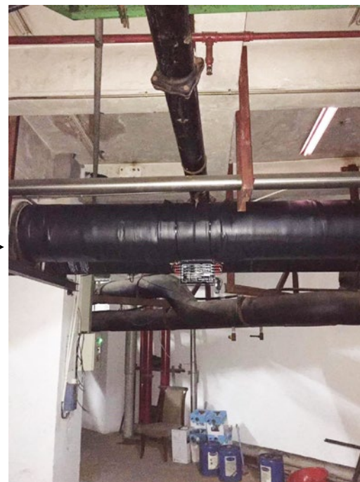
Step 2: Pipe is wrapped with insulation material, then install Vulcan S350 unit
