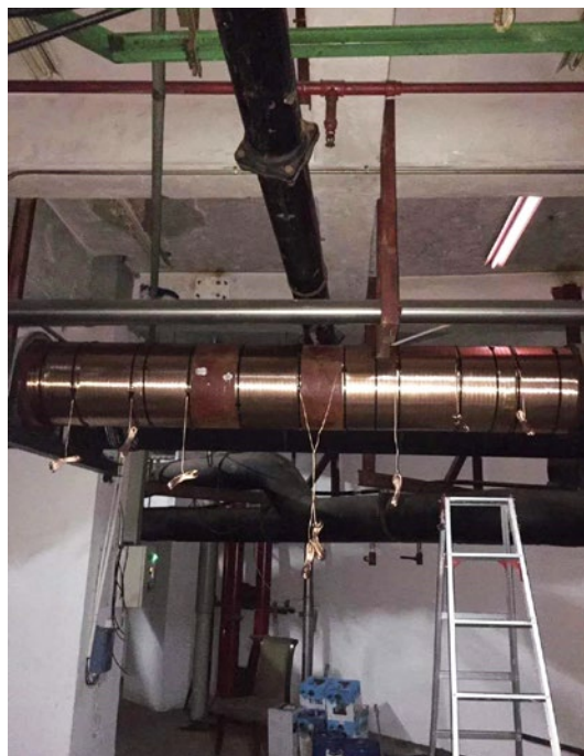
Step 1: Install the impulse bands
