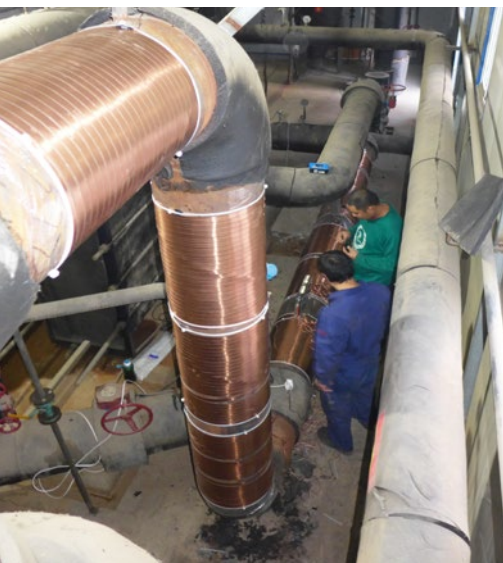
Vulcan S500 was installed in the heat exchange station.
