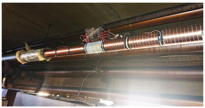
Vulcan S100 was installed on the main inlet to solve the scaling problems of the cooking and smoking chambers. The pipe insulation was removed to install impulse bands.
