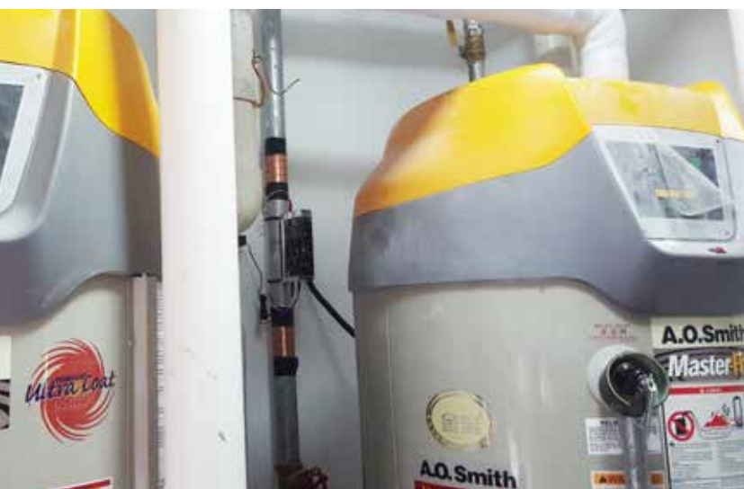
Vulcan S10 treats the living hot water for the office area.
