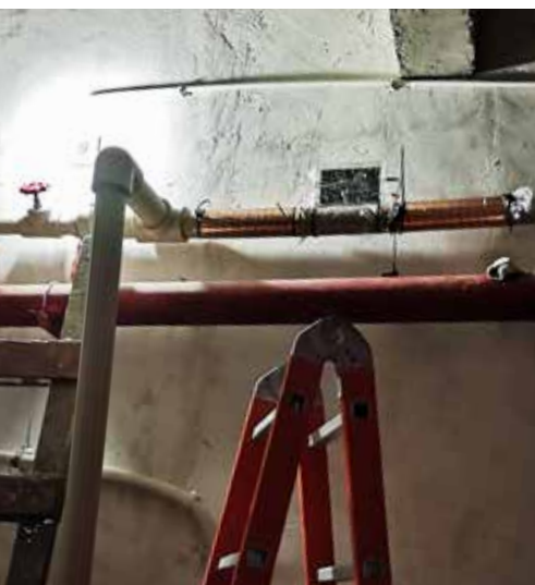
Vulcan S10 was installed in the hotel water main.
