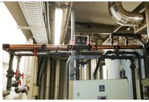
Vulcan S25 was installed on the main inlet to treat the cooling towers.
