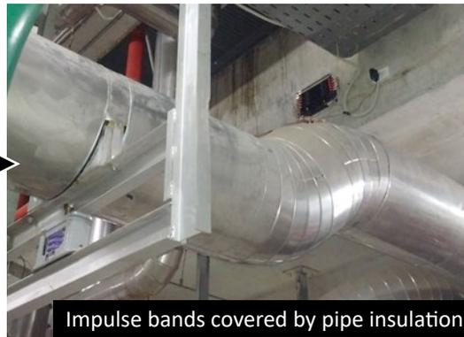
Impulse bands covered by pipe insulation
