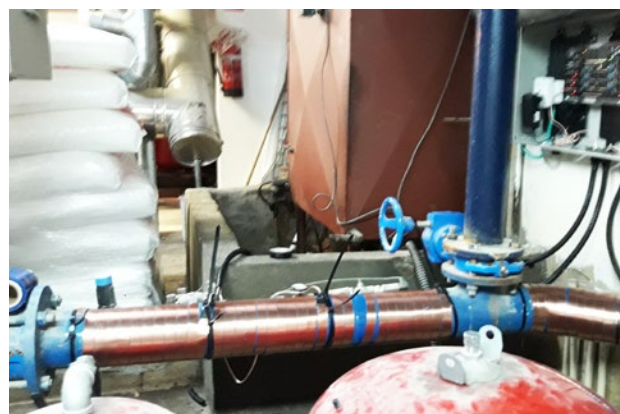
The salt bags on the left side are no longer used and replaced with Vulcan.
