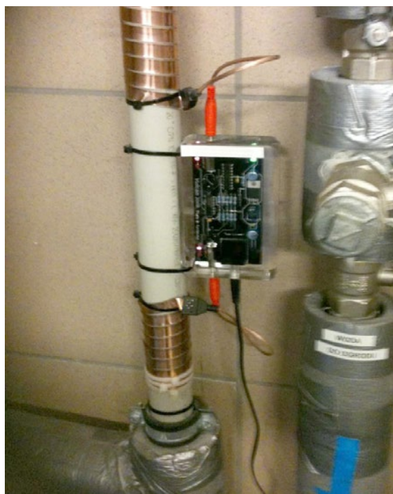
Installation of the Vulcan unit
