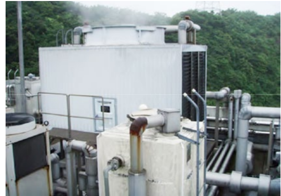
The cooling tower roof of medicine factory
