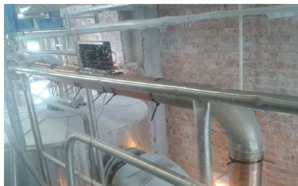
Installation of Vulcan S100 on lime kiln
