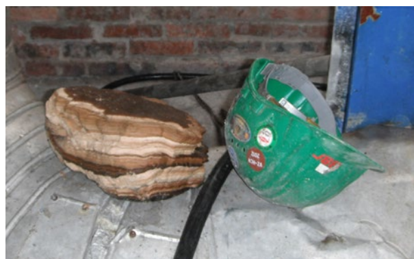
Deposit removed from pipe after Vulcan installation
