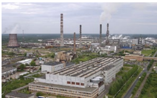
Mondi Štětí a.s manufacturing plant in the Czech Republic
