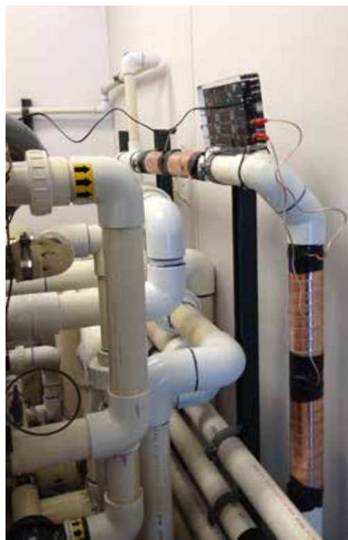
Vulcan S25 installed for the Spa water treatment
