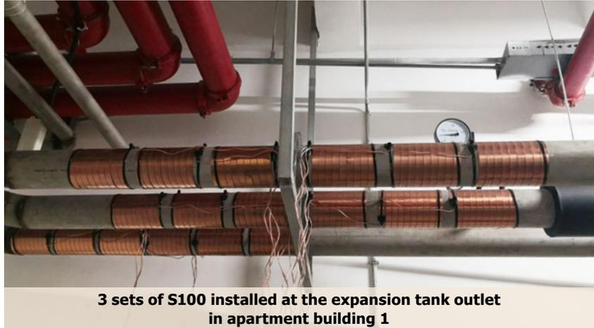
3 sets of S100 installed at the expansion tank outlet in apartment building 1
