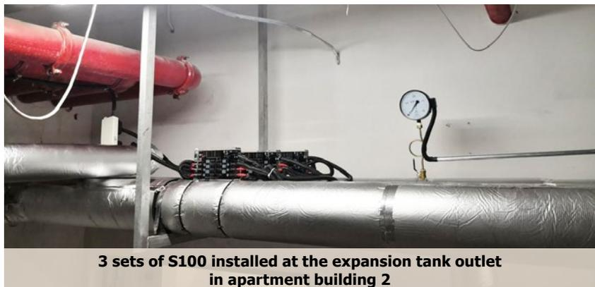
3 sets of S100 installed at the expansion tank outlet in apartment building 2
