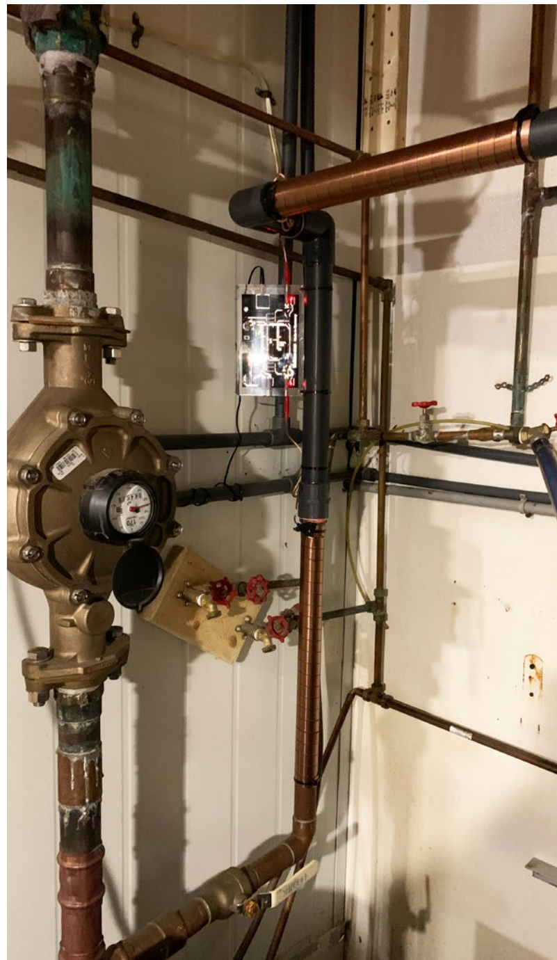
Vulcan S10 was installed to treat the whole piping systems.
