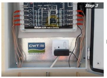
Connect the Vulcan S250 unit with the impulse bands. (Vulcan unit was installed in the outdoor case to prevent from humidity.)
