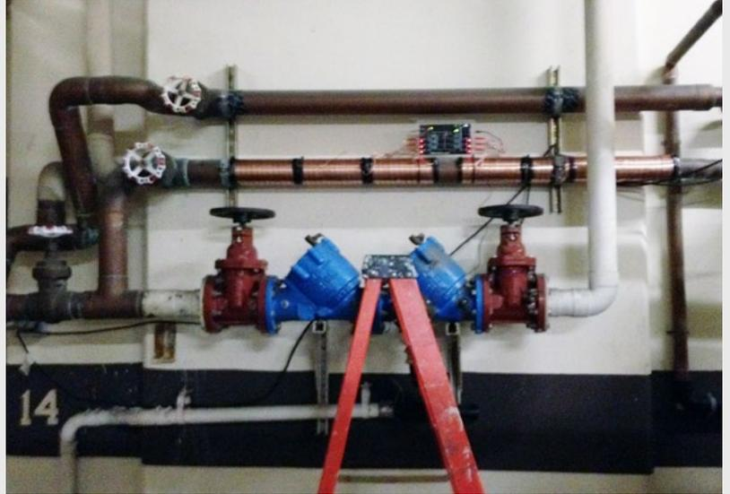
Vulcan S100 installed on the cleaning system
