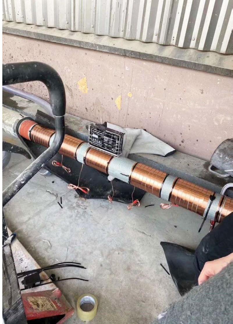
Remove the pipe insulation and install Vulcan S100.
