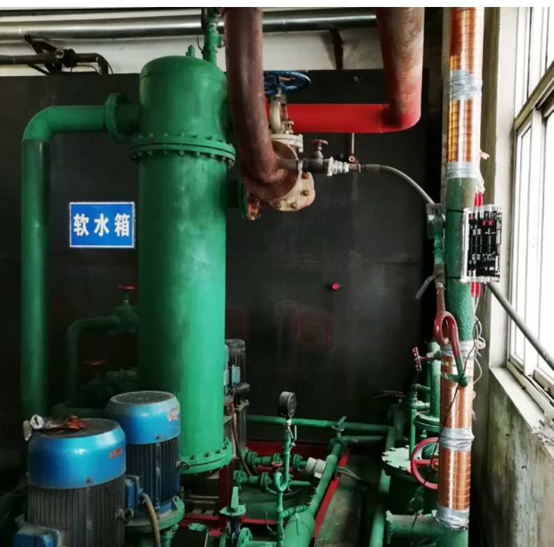
Vulcan S25 was installed on the main water pipe in the boiler room.
