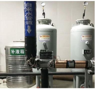
Vulcan S10 was installed in front of the heat exchanger to solve scaling problems in heat exchangers, pumps, water tanks, shower heads and the whole piping system.
