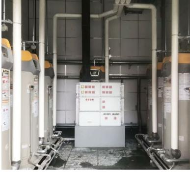
Both sides of the picture are water heaters, Vulcan S10 was installed in the water inlet of the heaters.
