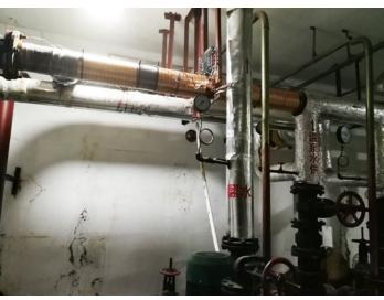
The hot spring water pipeline is far away from the villa, so the water has to pumped. Vulcan S150 was installed on the delivery pipe.
