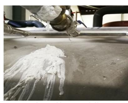
Hot spring water flows out of the pipe joint, it builds up stalactite-like scales over time.
