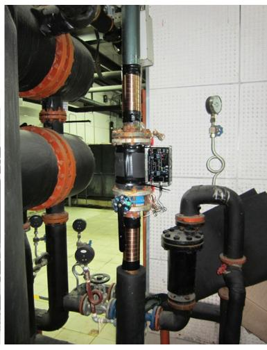
Another Vulcan S10 was also installed at the water inlet of the heat exchanger. The advantage of Vulcan: no chemical, no need to stop hot water supply.
