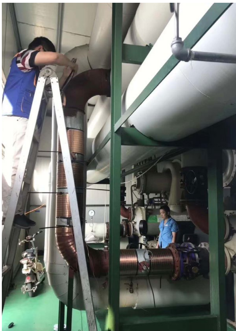
Vulcan S250 was installed on the main water pipe for the air conditioning cooling water.
