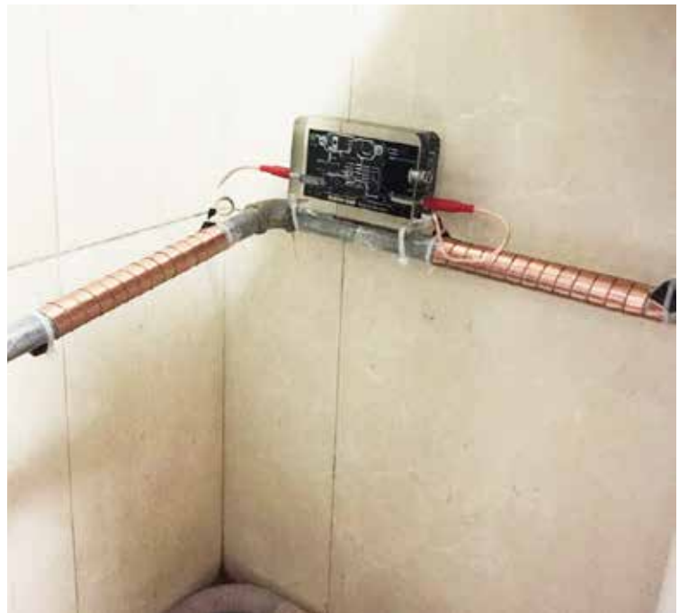
Vulcan 3000 installed on the smaller pipe in the dormitory
