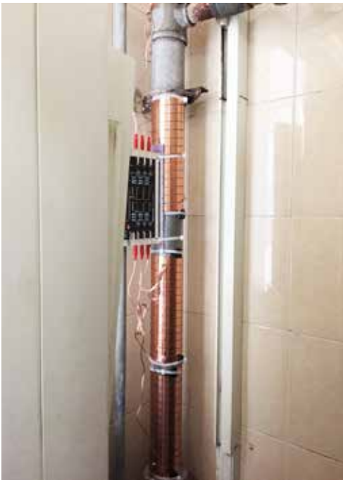
Vulcan S100 installed on the main water line
