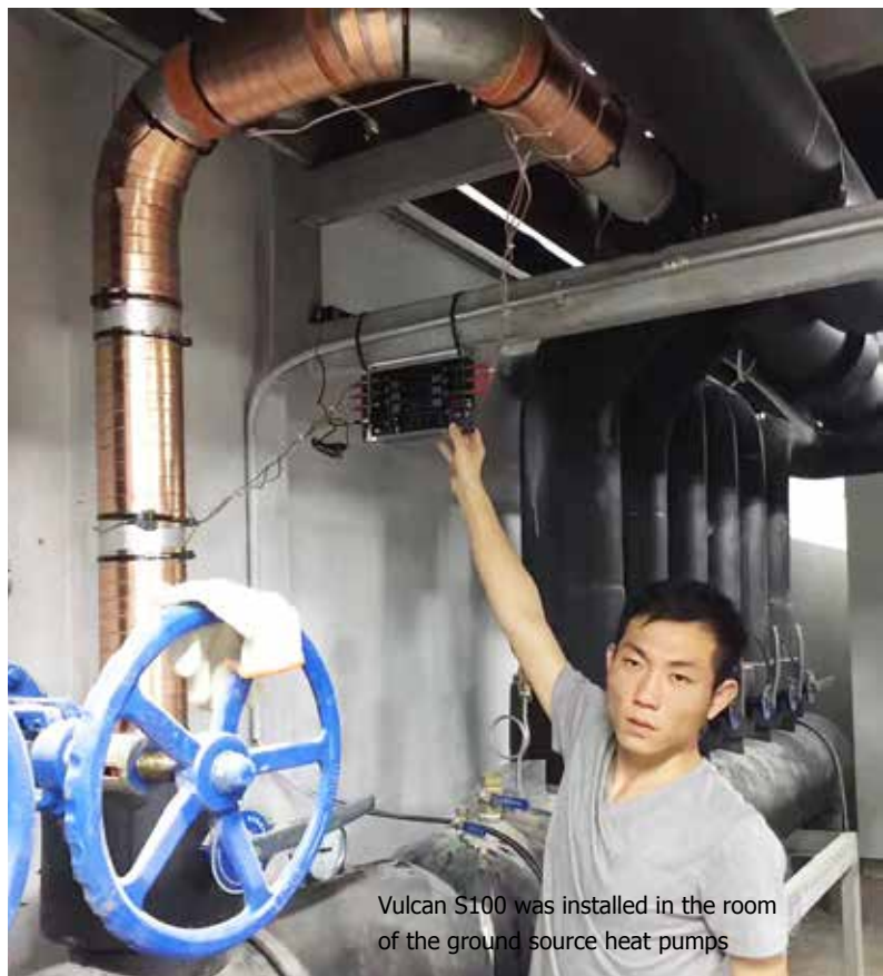
Vulcan S25 was installed in the room of the ground source heat pumps
