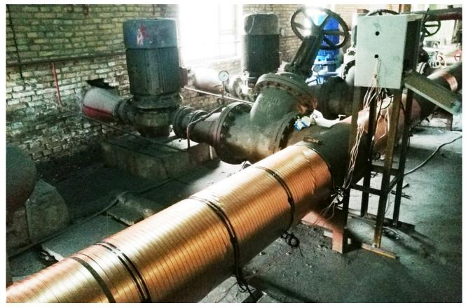
The Vulcan S500 solves the serious scaling problems in the circulating cooling water system, the water softener has been replaced.
