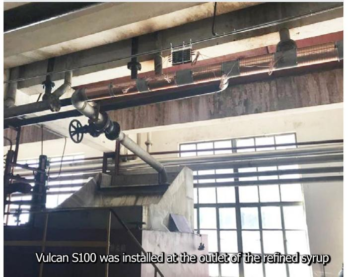
Vulcan S100 was installed at the outlet of the refined syrup
