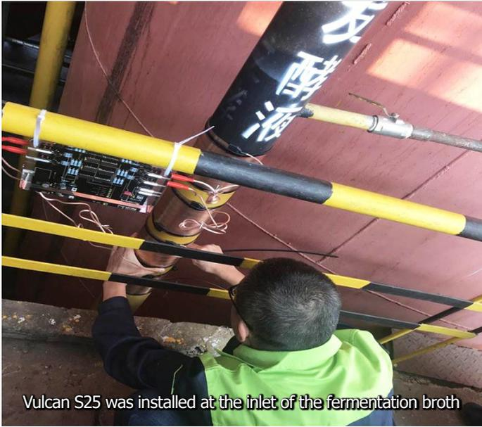
Vulcan S25 was installed at the inlet of the fermentation broth
