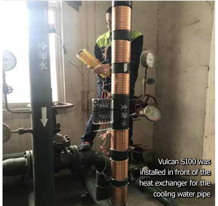
Vulcan S100 was installed in front of the heat exchanger for the cooling water pipe
