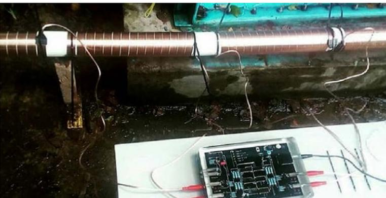
**Picture 1.** Vulcan installation process at the main incoming water line.
