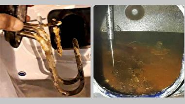
**Pictures 4 & 5.** Three weeks after Vulcan installation, initial scale has been eliminated.
