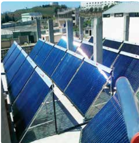
Solar heating panels of an apartment house
